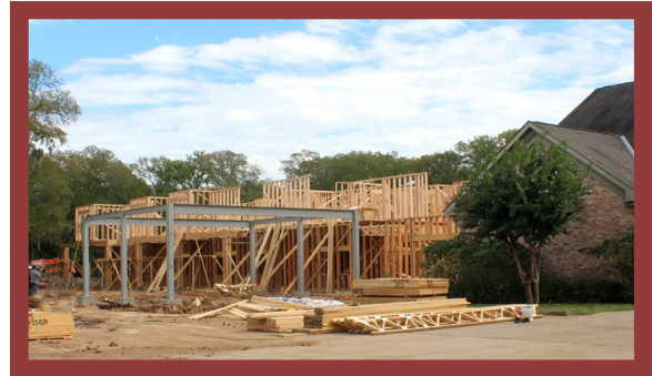
Steel Porte-cochere & Framing of Second Story Walls
